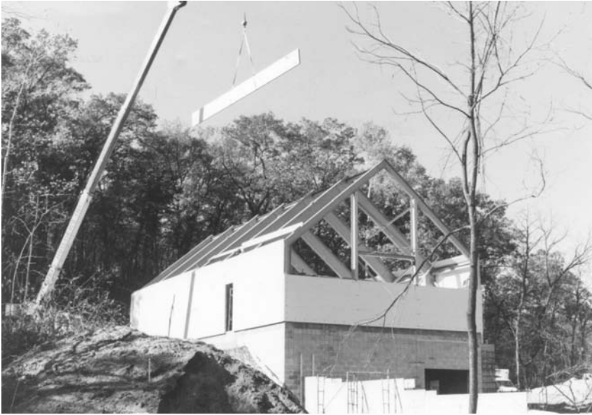
Fig. 48 All-composites skeleton. (Courtesy of Strongwell Company)
