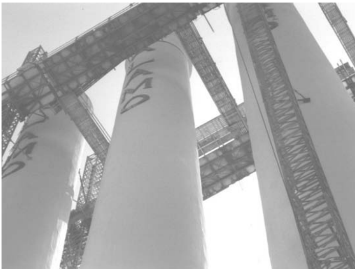
Fig. 9 Structural strengthening of chimneys using polymer composites. (Courtesy of Fyfe Co. LLC)
