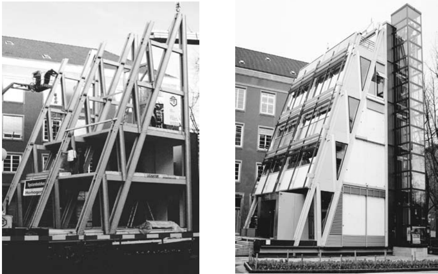
Fig. 46 All-composite "Eyecatcher" building in Switzerland: (a) pultruded frame skeletons and (b) the completed structure. (Courtesy of Fiberline Composites A/S)
