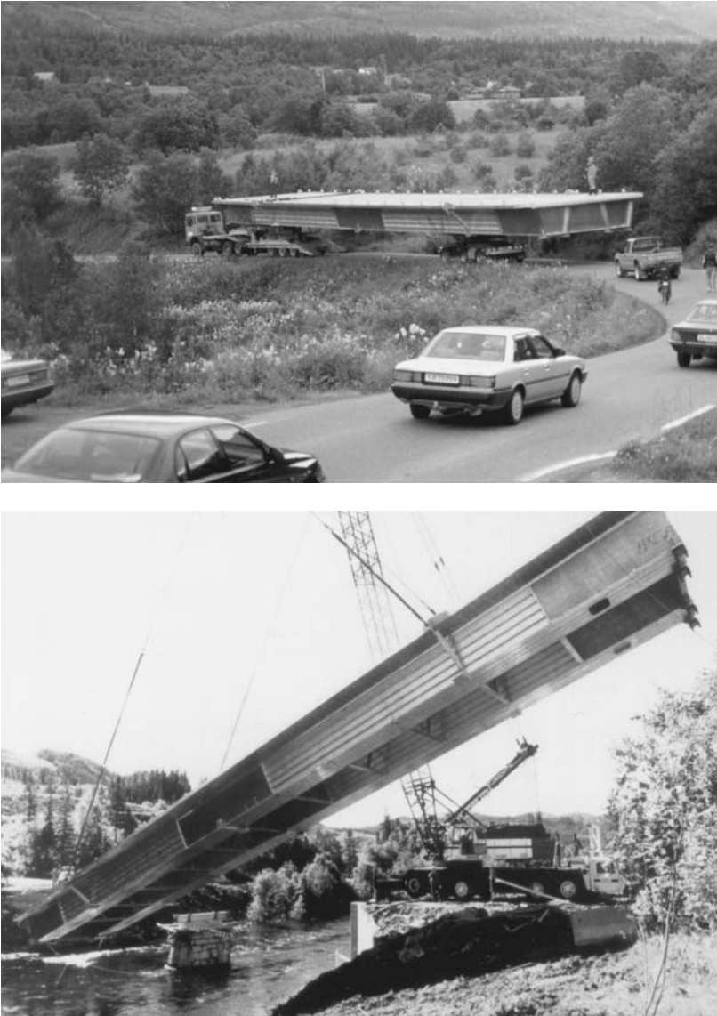
Fig. 9 The Foresmo bridge in northern Norway is an excellent example of the use of Al-Mg alloys for built-up girder systems; these photos illustrate a major advantage of replacement aluminum bridges: the ability to prefabricate the spans, (a) transport them, and (b) erect them in place quickly, minimizing the disruption to traffic.
