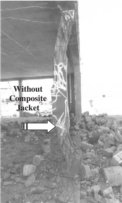
Fig. 18 Blast-resistance enhancement of reinforced concrete structures. [Courtesy of Structural Composites Construction Inc. (SCCI)]
