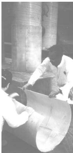
Fig. 23 Hard shell precured composite retrofit system. (Courtesy of Professor M. Haroun, University of California, Irvine)
